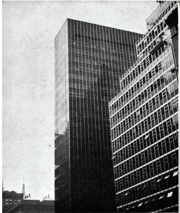
Figura 7. Lever House de Skidmore, Owings y Merrill
